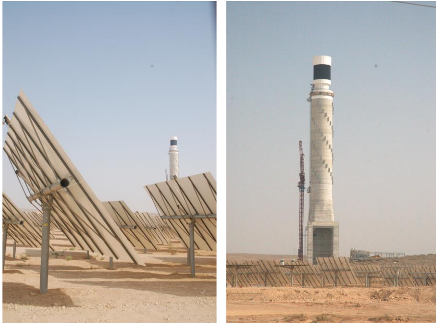
Ashalim Concentrted Solar Power Plant
