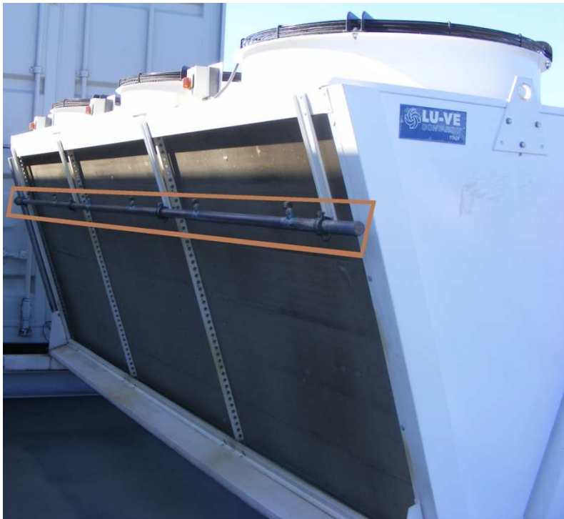
Image 21 - Dry cooler installed in Dunakeszi Tesco supermarket with a water spray system (11)
