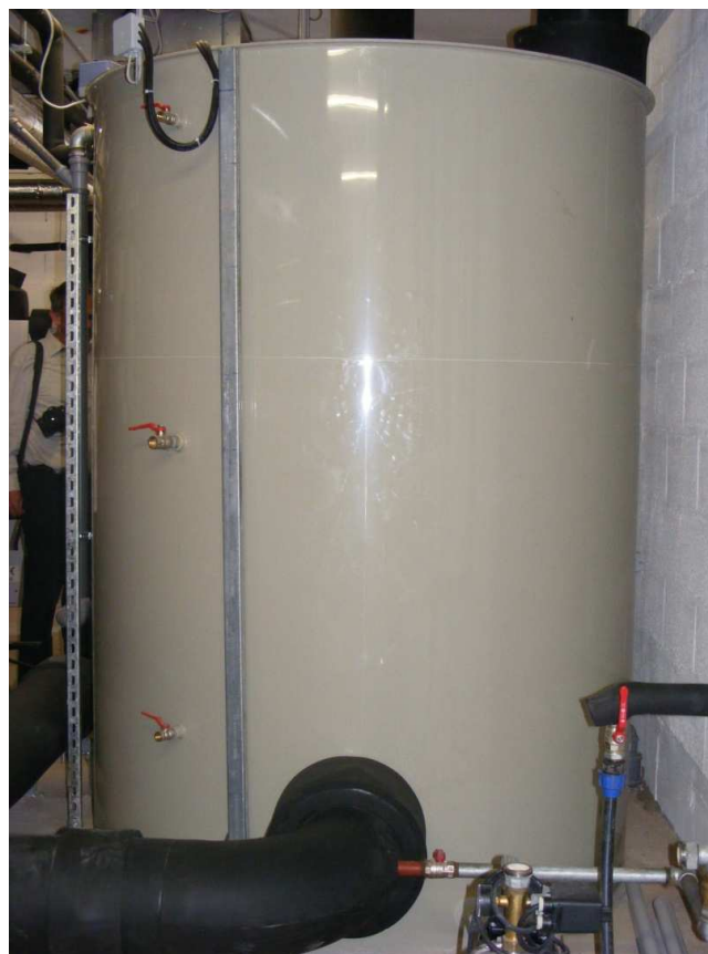
Image 18 - Heat container used in Dunakeszi Tesco supermarket (11)
