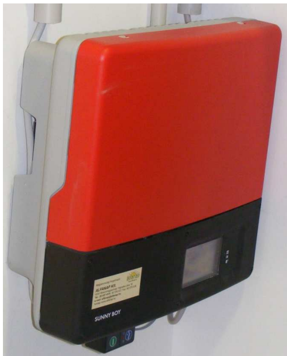
Image 26 - Sunny Boy inverter used in Dunakeszi Tesco Supermarket (11)
