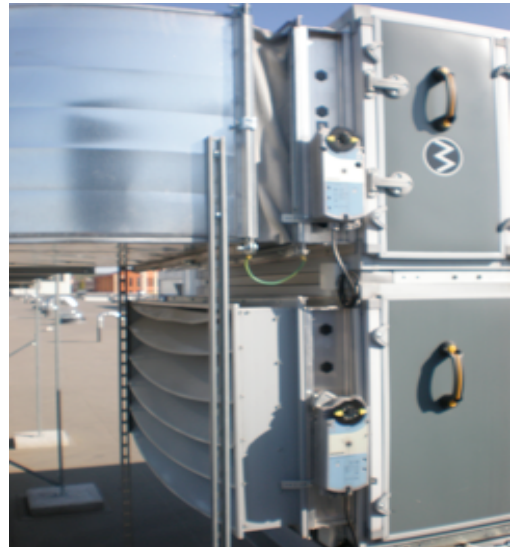
Fig. 7.37 Details of heat recuperator
