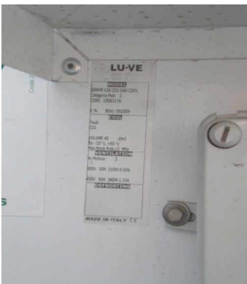
Fig. 7.4 Plate of characteristics
