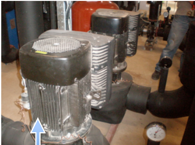
Fig. 7.32 Details of compressors
