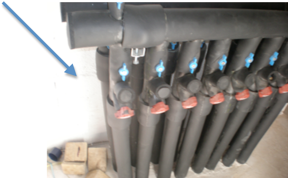
Fig. 7.35 Pipes system to ground
