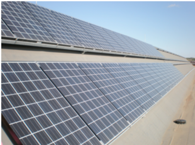
Fig. 7.23 Set of solar panels 45°
