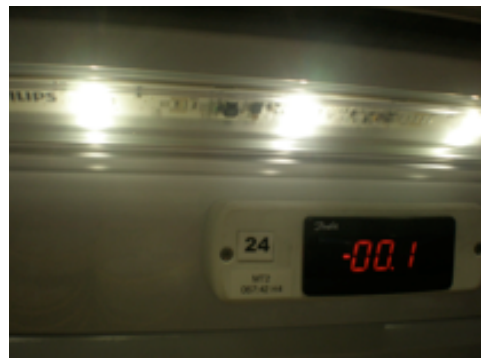
Fig. 7.38 Leds in refrigerator cabins
