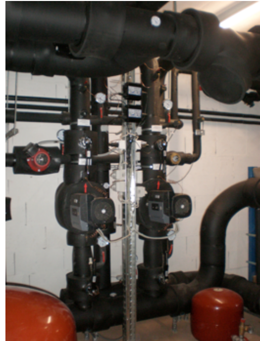
Fig. 7.31 Details of compressors 2
