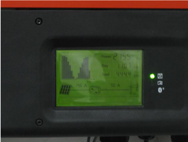
Sunnyboy Solar inverters
