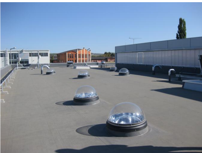
Light domes on the rooftop
