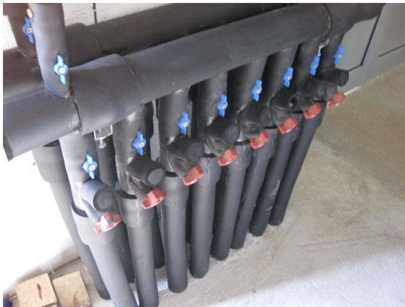
Pipes which go in to the ground
