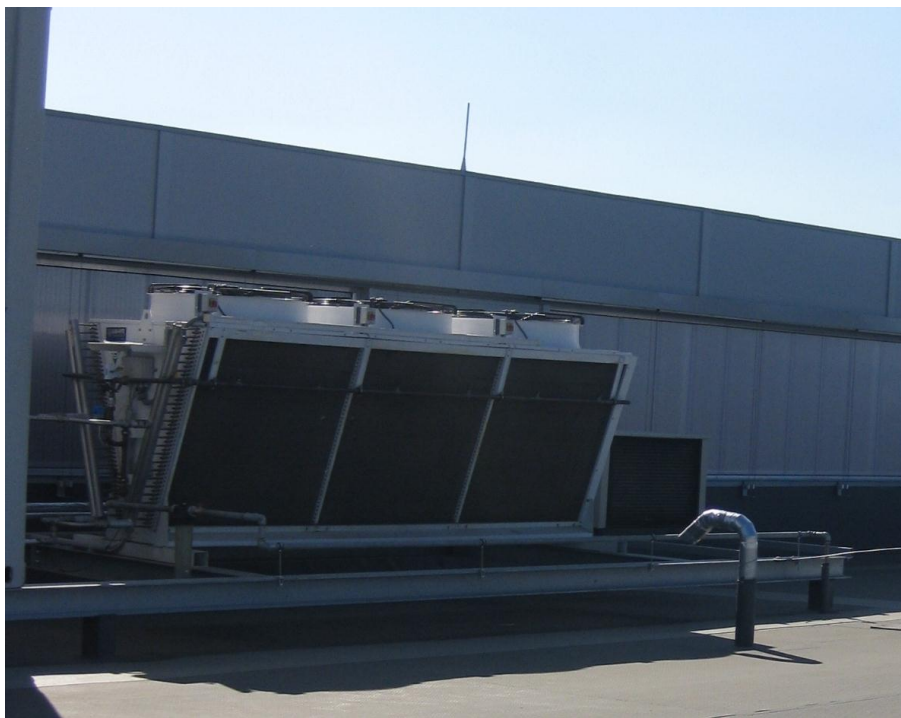
Condenser of the rooftop
