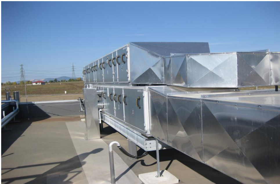
The heat exchanger in series on the rooftop
