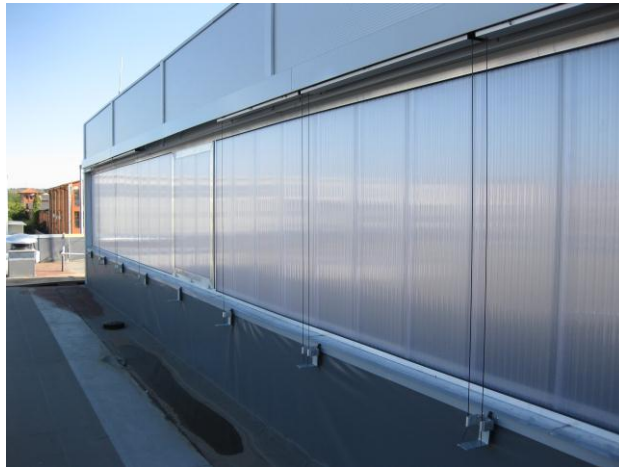
Blinds on the roof of the building
