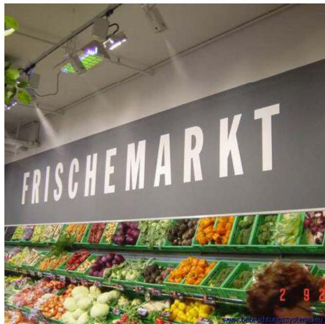
Air Humidification in supermarket
