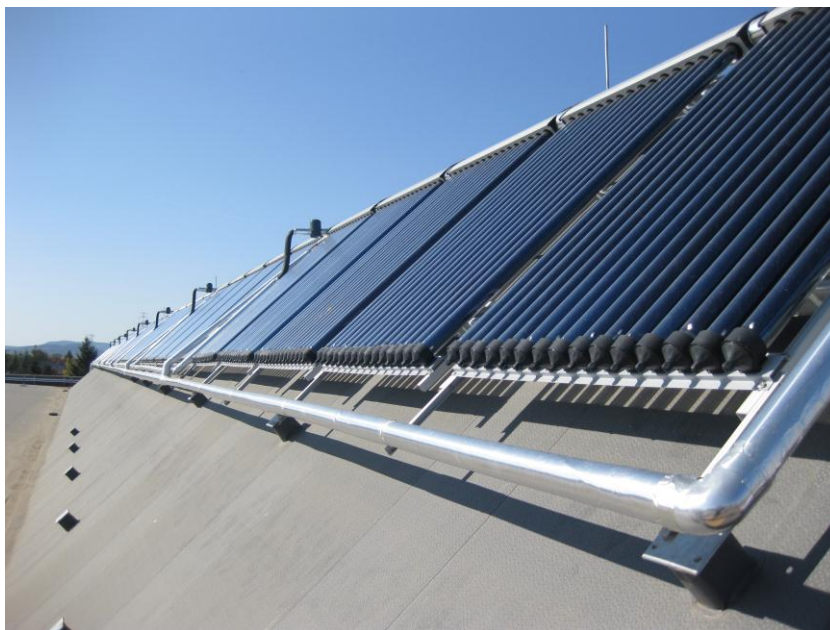
Evacuated tube collectors
